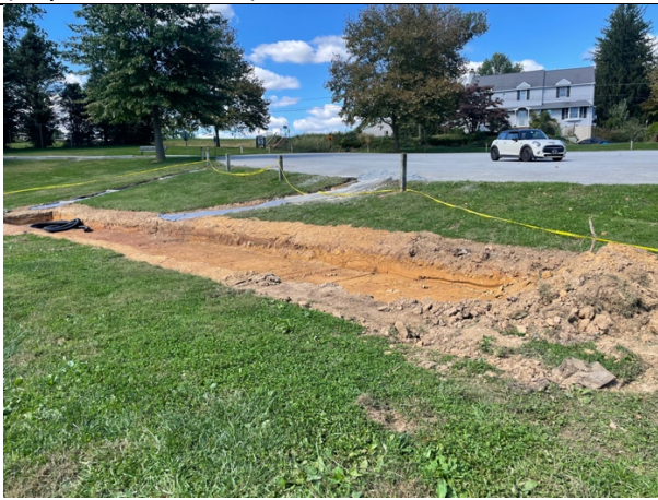
Construction Days 3&4 (base dug out and leveled)
