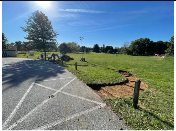
Construction Days 1&2 – inlets to garden built
