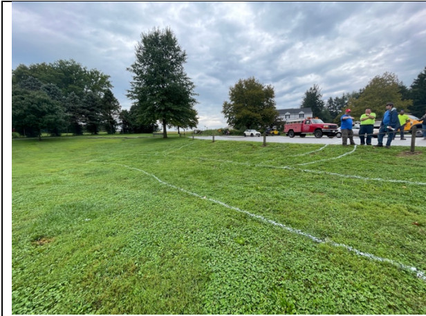
Harmony Park Before Construction (September 2021)
