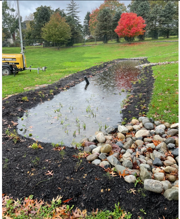
Test 1: 2"+ rain event 10/26/2021 – 5 hours after storm event ended
