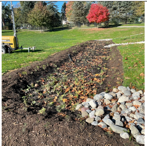
Test 1: 2"+ rain event 10/28/2021 – 48 hours after storm event ended – fully drained.
